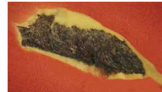
Paint peeling surface (350x)
